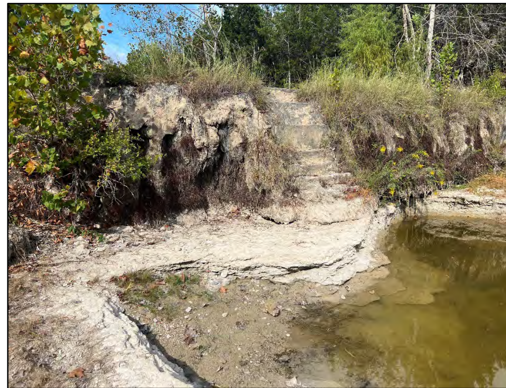
Photo 8: Stairs leading to top of historic dam.
