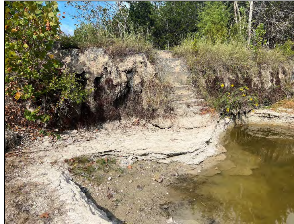
Photo 8: Stairs leading to top of historic dam.
