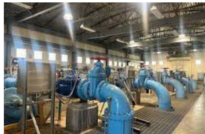
Figure 11. West Travis County PUA Facility
