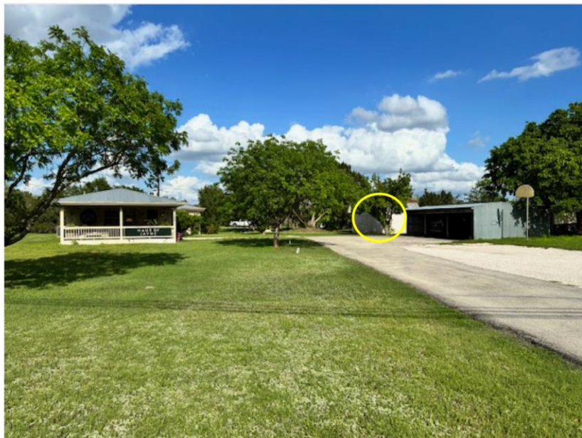
766 Old Fitzhugh Shed: “Current Conditions, view from Old Fitzhugh Rd”. Applicant image, 2026
