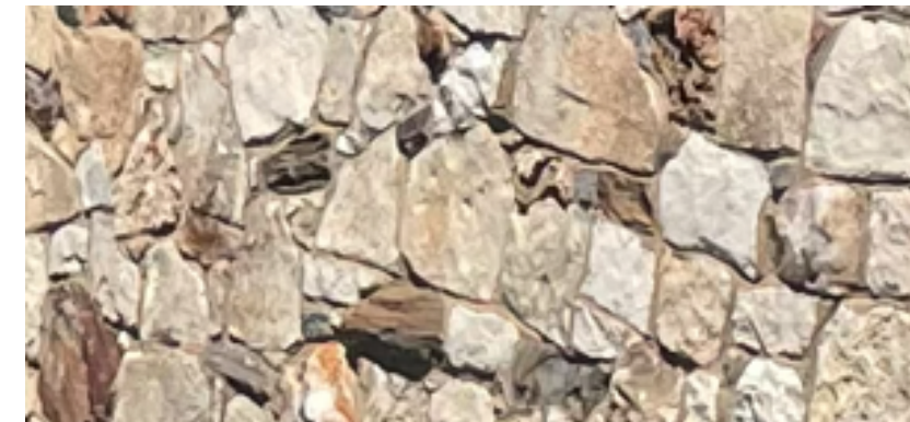
EXISTING MASONRY TO REMAIN
