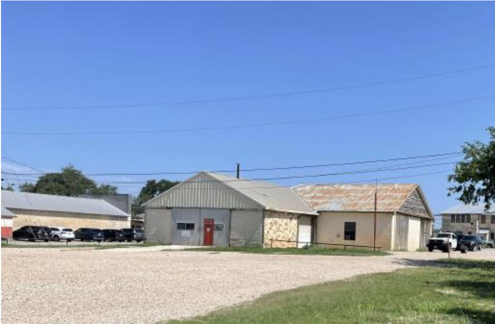
“Current Conditions, view from interior/ rear parking lot”. Applicant image, 2026
