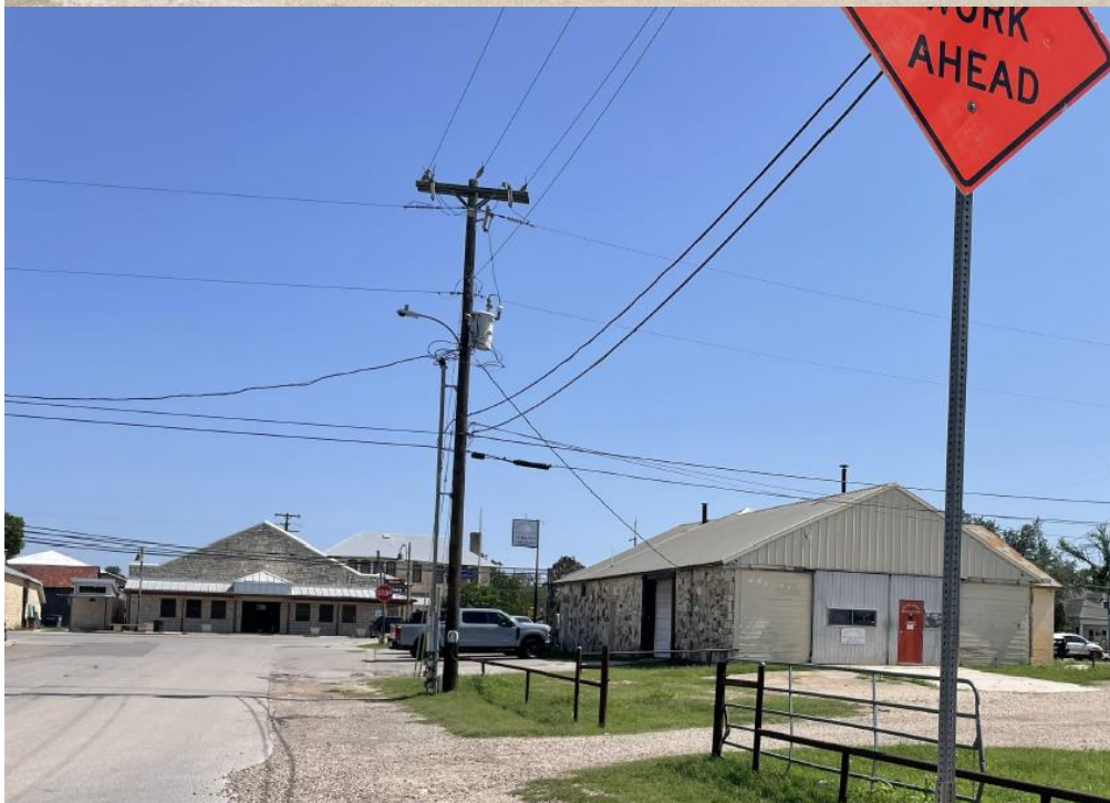
“Current Conditions, view from College St”. Applicant image, 2026 and Google Maps image.
