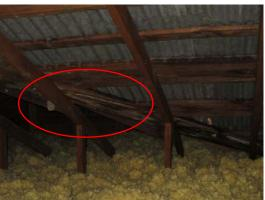
**Flashing missing**: There doesn't appear to be any counter flashing at the roof wall connections at various locations. There is a possibility of water damage to the siding and framing where ever flashing is missing.
