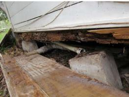
**Under ventilated:** The ventilation under the house does not appear to meet modern ventilation requirements. Lack of proper ventilation can contribute to excessive moisture in the crawl space which can be conducive for mold, termites and other problems. There should be a minimum of 1 square foot of ventilation per 150 square feet of crawl space.
