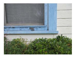
Windows in poor condition: The windows are older wood frame windows which appear to be in poor condition. Windows are damaged, leaky and drafty. In addition, the glass in some of the windows is loose and some wood rot was observed.
