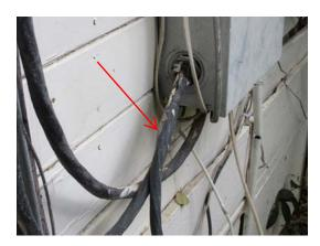
**Arc fault missing:** This home does not meet modern electrical standards regarding AFCI (Arc Fault Circuit Interrupter) protection on some of the circuits/breakers.
