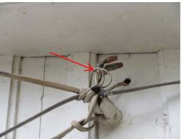
**Switch not approved for exterior:** The light switch at the patio exterior is not approved for exterior use. Recommend changing out the switch/cover for a weatherproof switch or cover.
