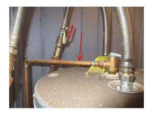
**Piping not insulated:** The water lines at the water heater are not insulated. Installing pipe insulation can help improve efficiency.
