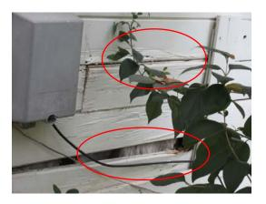
**Foliage touching house:** There is foliage in contact with the structure at some locations around the exterior. This is considered a conducive condition for carpenter ants which are a wood destroying insect. I recommend trimming back all foliage at least 12 inches. Foliage prevented visibility of various exterior walls and the foundation in some areas. Inspection of areas obscured by heavy foliage is very limited.
