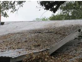
**Possible roof leak:** There appears to be evidence of a roof leak at the left back roof slope over master bathroom. Water evidence was observed at the bathroom ceiling. Recommend confirmation by a roofing contractor and repair as necessary.
