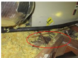
Air loss at coils: There is loss of conditioned air at the areas where the refrigerant lines and condensate drain lines exit the evaporator coils (at furnace/air handler). Recommend having these areas sealed.
