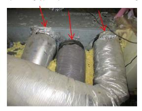
**Insulation pieces in registers:** There appears to be insulation pieces in the registers at various locations. This may be an indication of damage to ducting.
