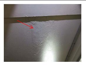
**Possible mold like substance:** There appears to be a mold like substance on the interior walls at master bathroom (sink cabinet). This appears to have been caused by a current moisture or water issue possible due to leaks at this area. All water damaged or mold damaged drywall should be removed.
