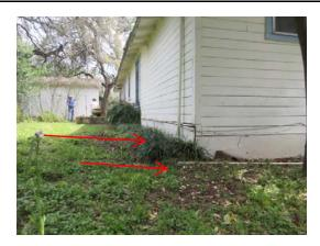
**Water pooling:** There are low areas at various locations around the foundation perimeter where water may be pooling when it rains. In some cases expansion and contraction of soils around the foundation can cause foundation issues.
