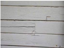
**Seal openings in walls:** Recommend sealing all openings or gaps in the exterior walls to prevent water intrusion and damage. Areas that should be sealed include: light fixtures, plumbing pipes, and around electrical panels. Also there are may gaps at siding and trim areas that need to be sealed. Because there are many unsealed areas, the walls may be subject to water intrusion under heavy rains. Some historic water damage may be concealed at some areas.
