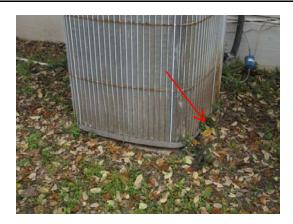
**Fins are damaged**: The AC compressor fins are bent and damaged. This does not appear to be effecting performance at this time.
