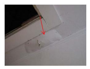
**Ceiling damage**: The ceiling appears to be have some damaged at the front right bedroom that may have been caused by water and/or termites.
