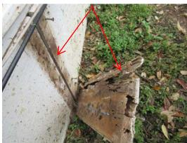
**Crawlspace access:** The foundation crawlspace does not have a proper access door or panel. There should be an operable door a minimum of 18 inches high and 24 inches wide, with a latch and handle.
