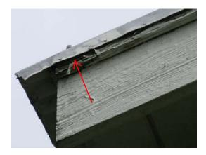
**Fascias water damaged**: The roof fascia boards are water damaged at some locations. Recommend replacement of water damaged wood, and recommend caulking and painting fascias as necessary.
