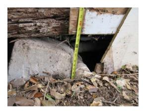
**Termite damage:** Evidence of a previous termite damage has been observed at some areas around the perimeter. See left side of foundation skirting for example. It is impossible to determine the extent of any structural damaged without removal of material to view the interior of the effected areas. If you are concerned about damage, I recommend opening this area and having the damage evaluated by a qualified contractor and repair as necessary.
