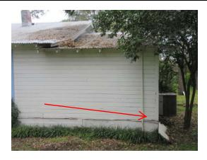
**Siding damage:** Siding shows signs of damage and is loose in one area at the left side of the house.
