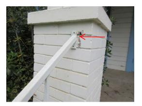
Cracking at patio: Cracking and general settlement was observed at the front patio.
