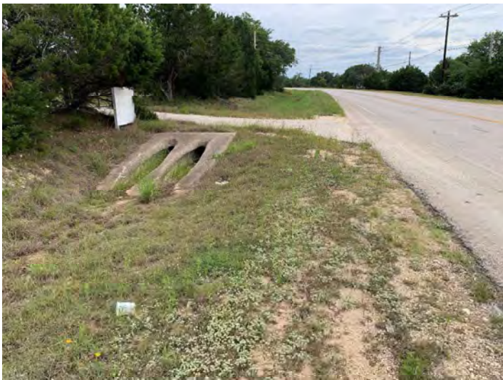
Photo 1: Front slope at existing driveway culvert north of Open Sky Road; driveway will be regraded to be compliant with ADA guidelines.
