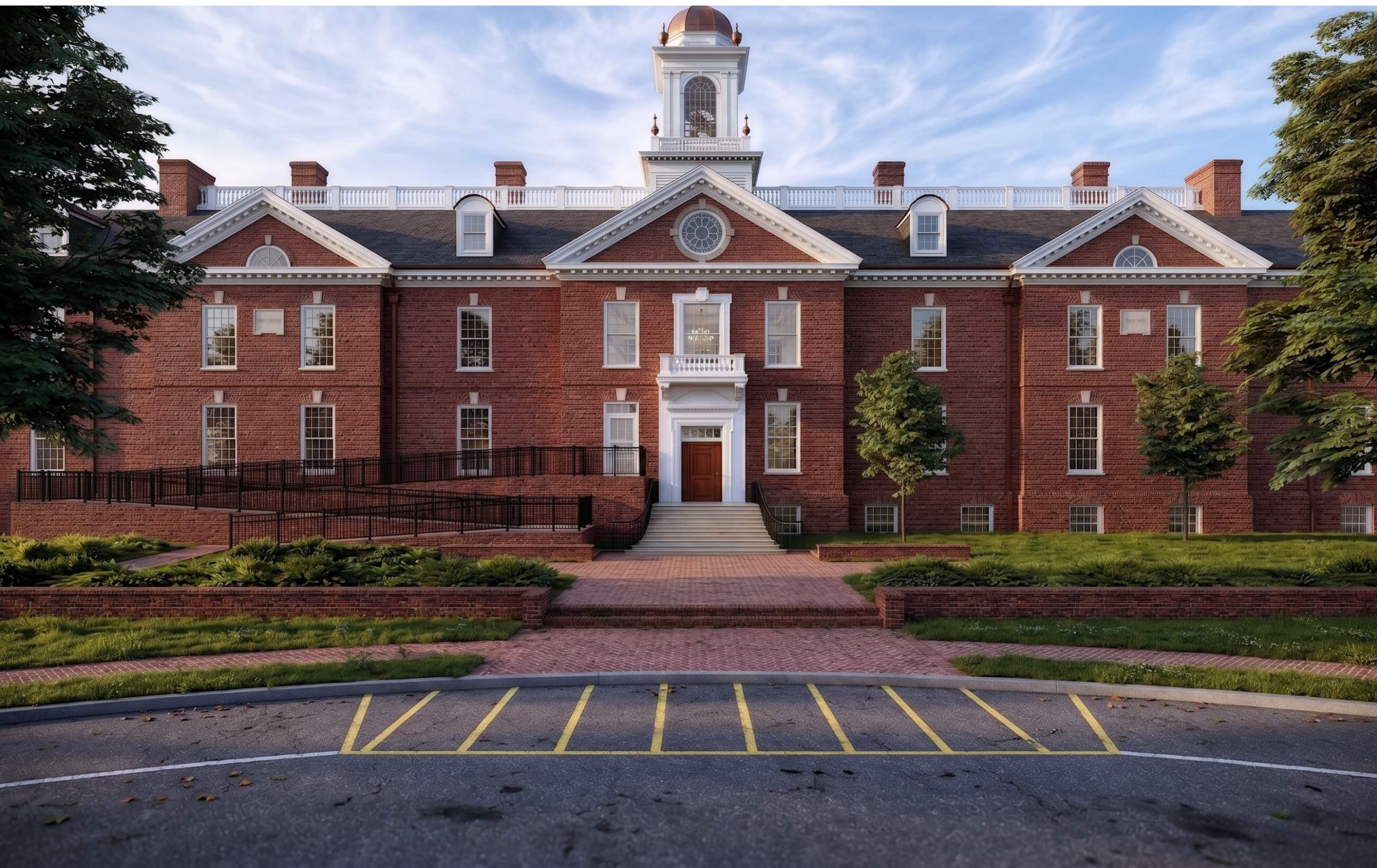
WEST ENTRANCE - VIEW FROM WEST
