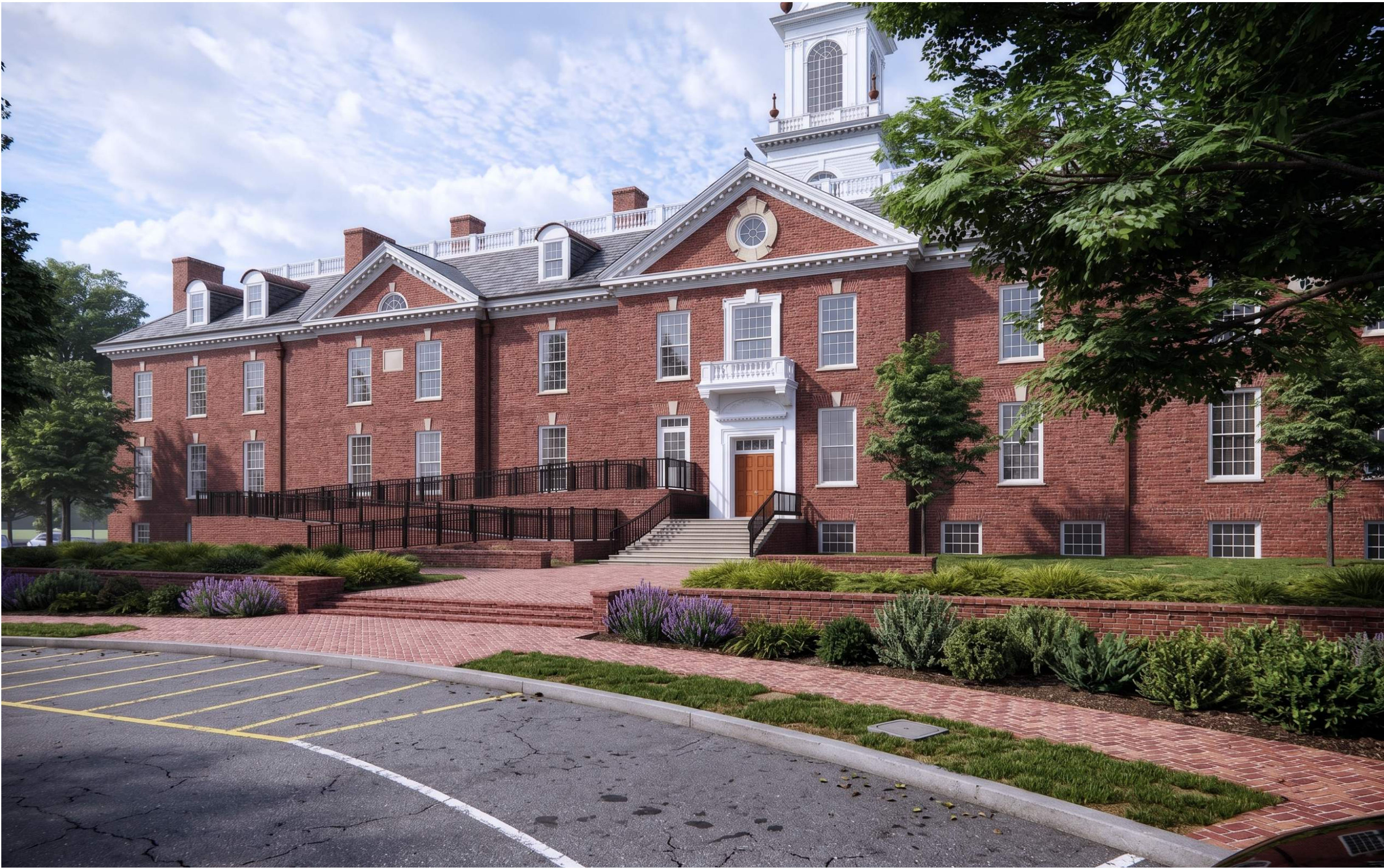
WEST ENTRANCE - VIEW FROM SOUTH
