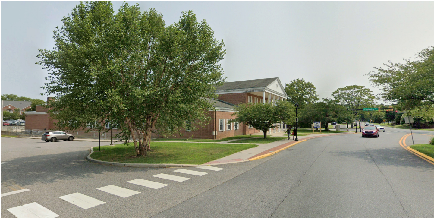
Library Entrance on Loockerman Plaza
