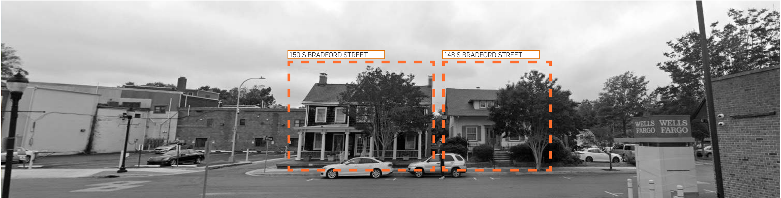
BRADFORD STREET, FACING WEST
