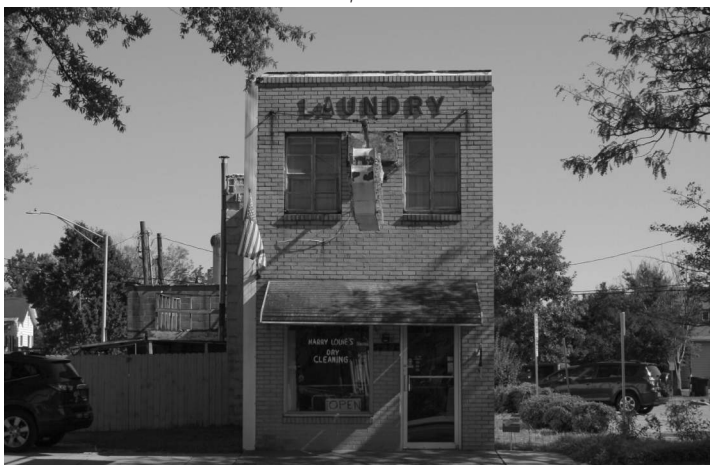
C: GOVERNORS AVENUE, NEIGHBORING BUILDING
