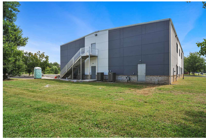
BUILDING - LEFT SIDE VIEW
