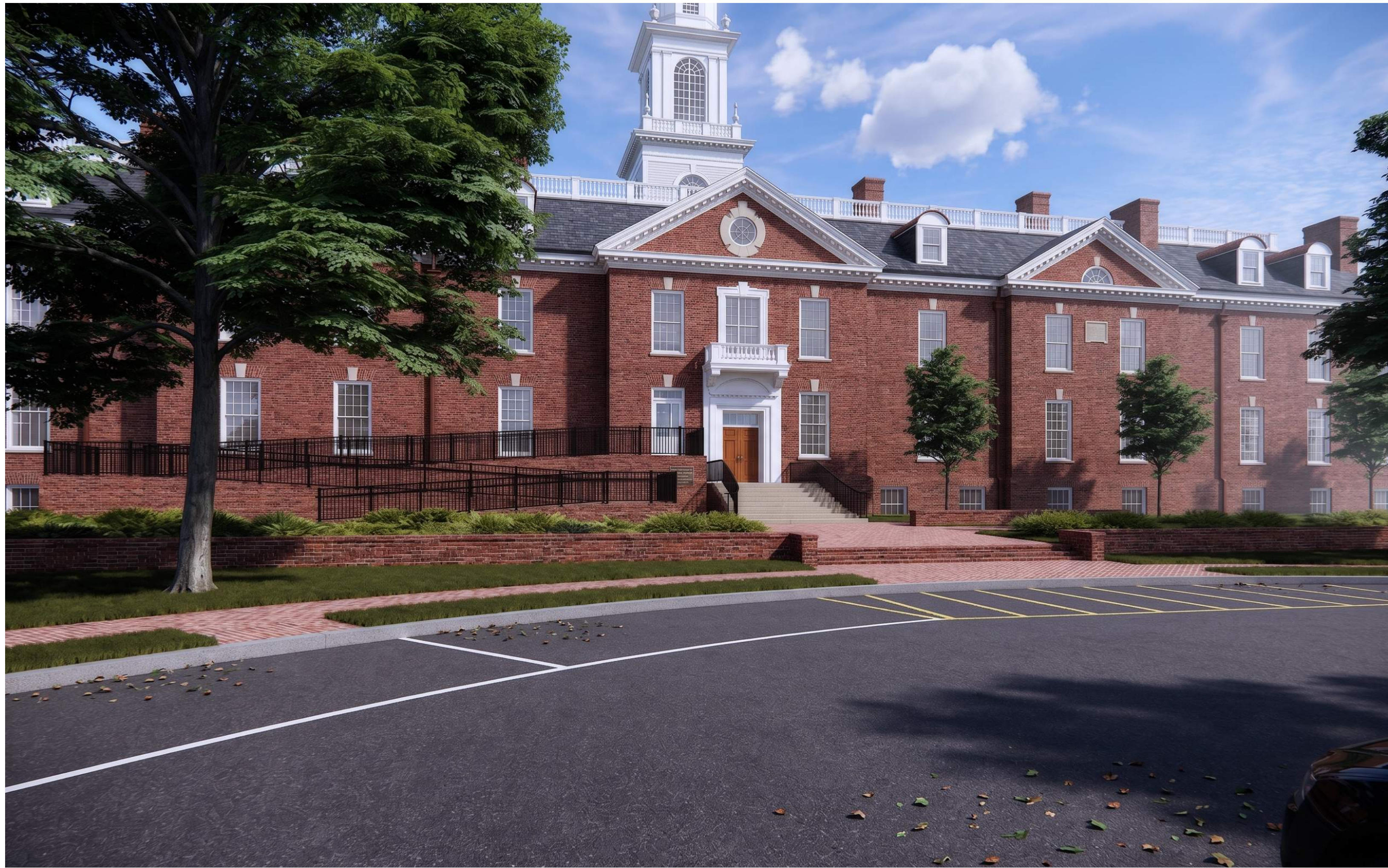
WEST ENTRANCE - VIEW FROM NORTH
