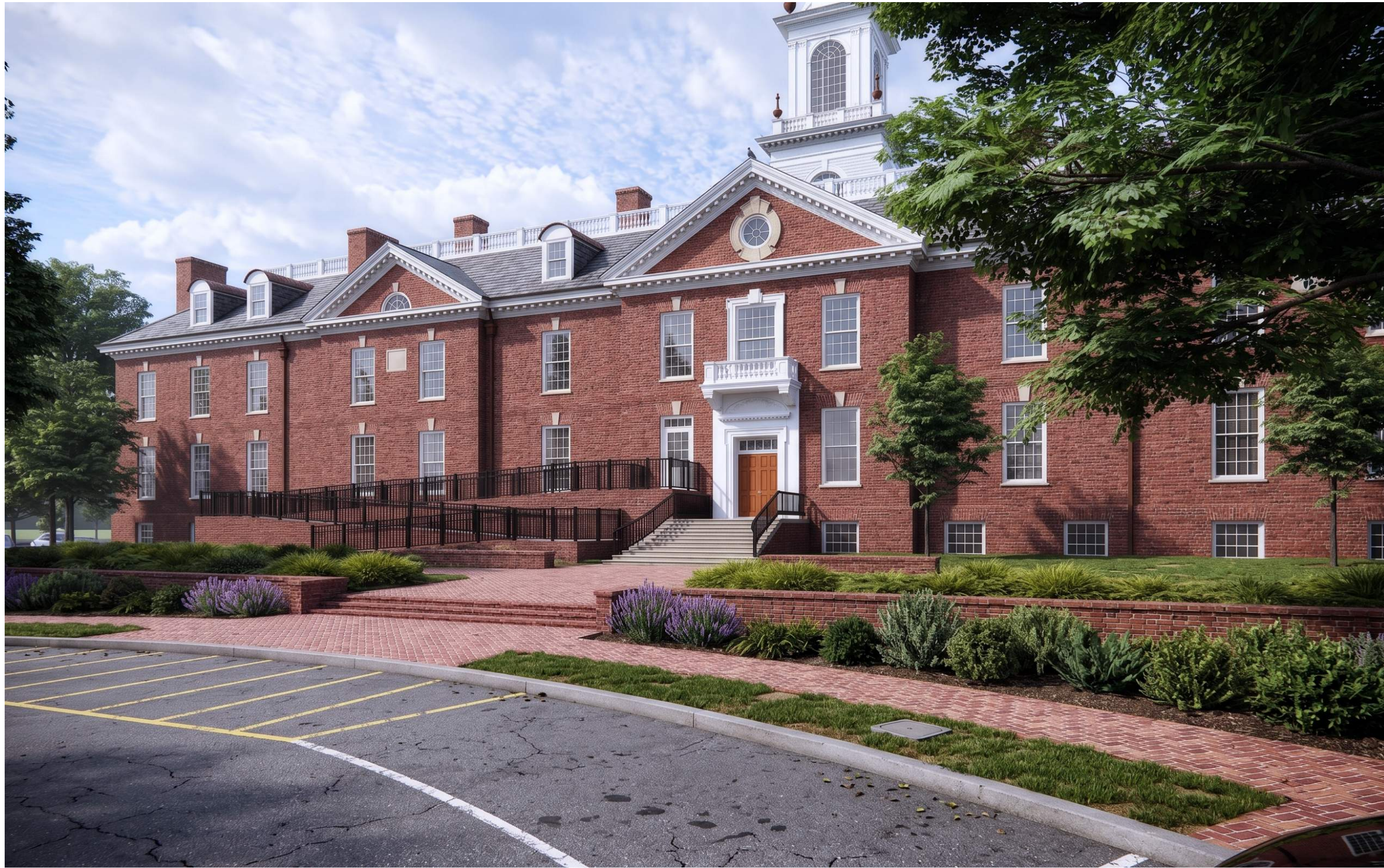
WEST ENTRANCE - VIEW FROM SOUTH
