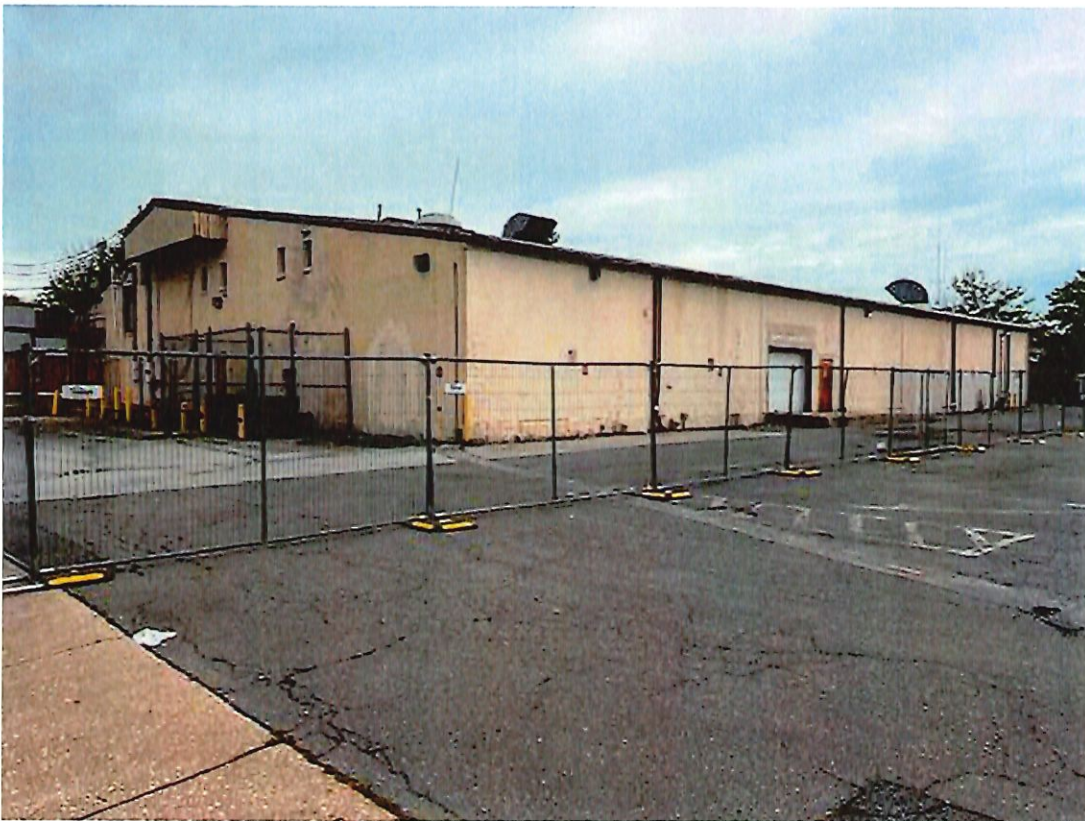
South-Facing Side of Property
