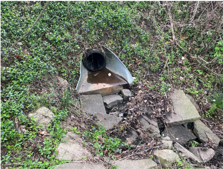
Blue Star Highway storm sewer drain outlet (12 inch)
