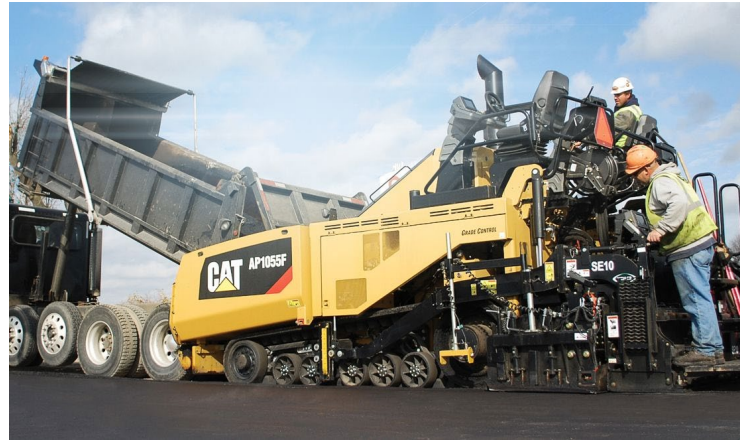
• Overlaying (Paving)
