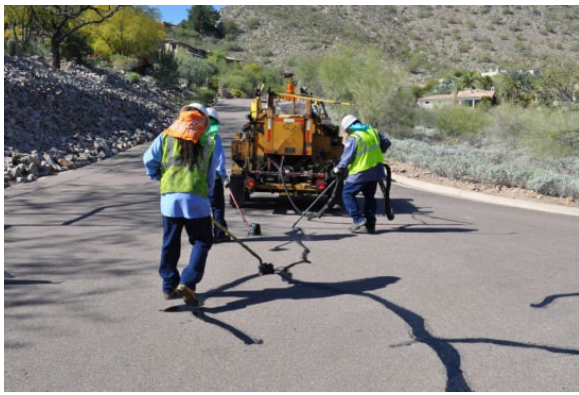
• Crack sealing
