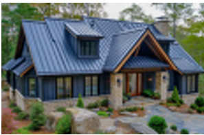
METAL ROOF STANDING SEAM [M1]
