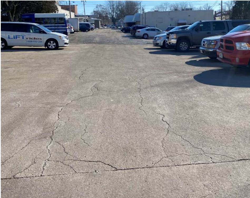
Photo 8: View of western side of west parking lot.
