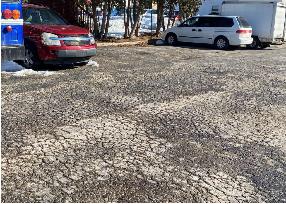
Photo 7: View of poor asphalt conditions in the west parking lot (east side of lot).
