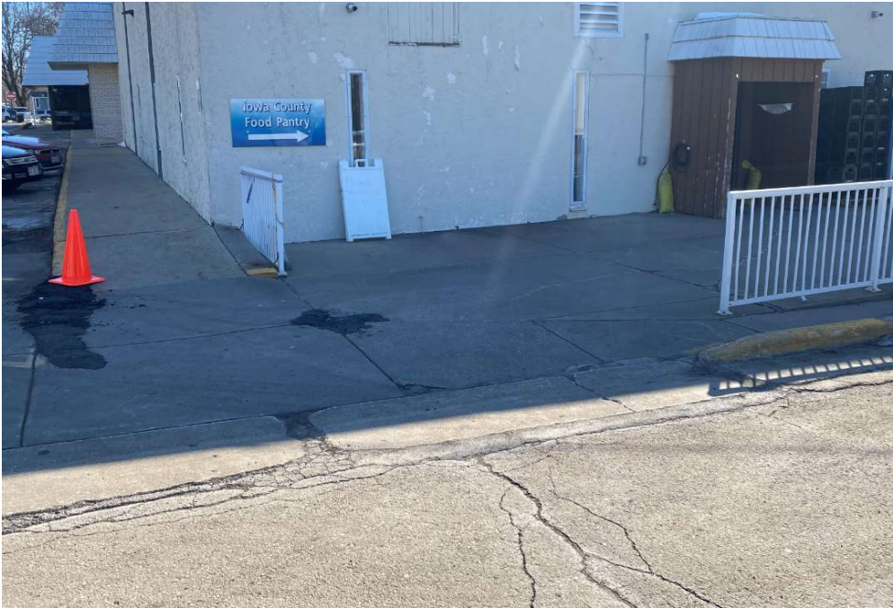
Photo 2: View of Concrete area looking East toward building.
