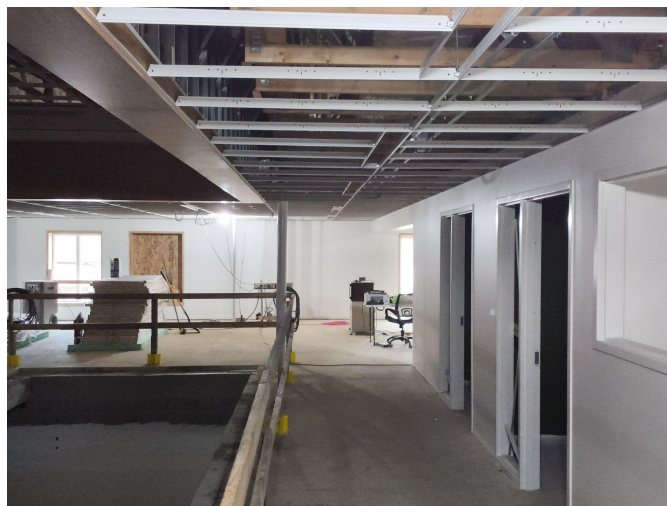
Original building - facing east
