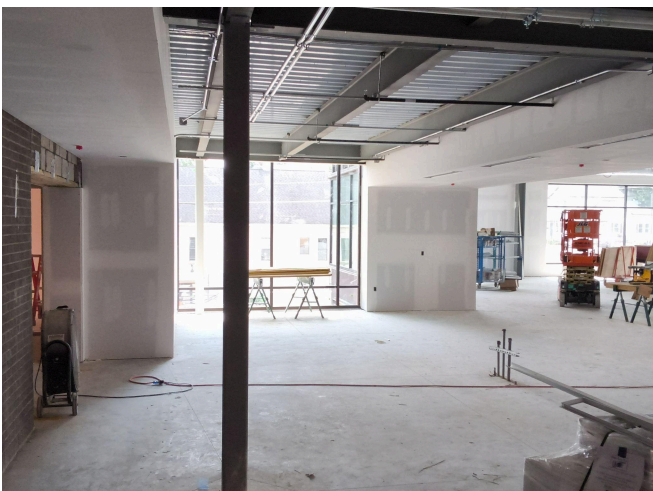
Addition looking south
