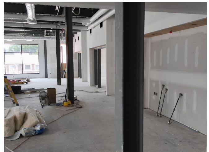
Addition looking west along community room
