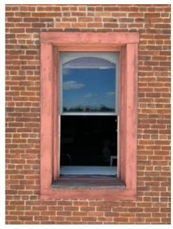
We would like to replace the window, sill and trim with a custom vinyl window from Tri-State Custom Windows. We will wrap the existing sill and trim in metal (and paint it the same color Burnt Red), or if possible, we would prefer to replace the wood trim and sill with Palight (in the same dimensions) also painted in the same color Burnt Red. The exterior color of the vinyl window itself would change to be Beige.
