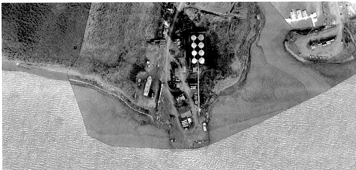
Figure 1: 2016 Aerial Photo of BAF Site
