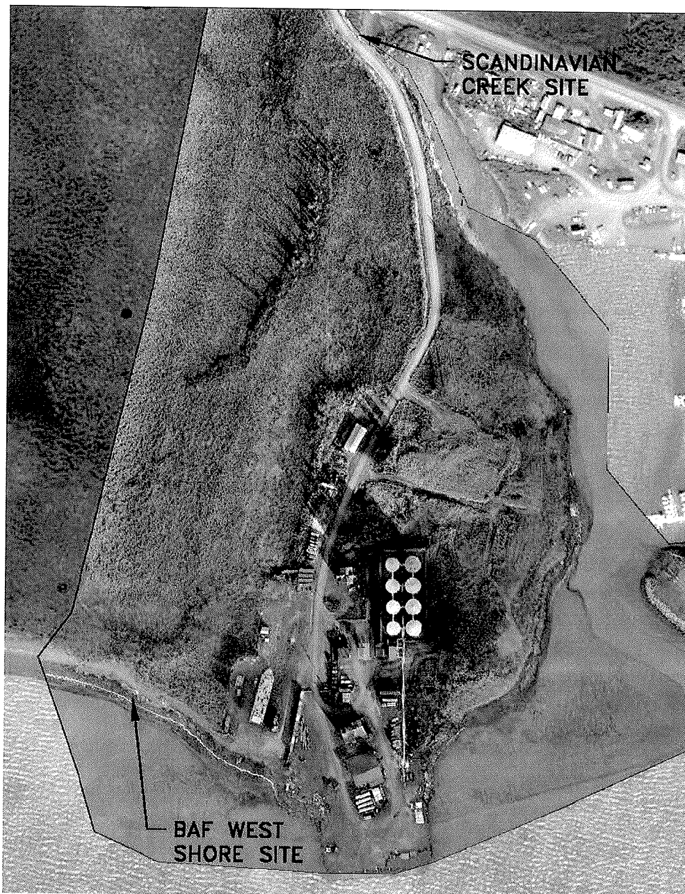
Figure 21: Other Erosion Protection Areas
