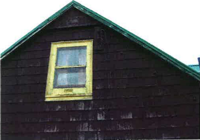
Upper Floor Windows
