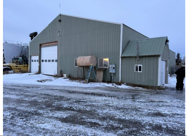
Overhead Door not Flush with Gravel Entry
