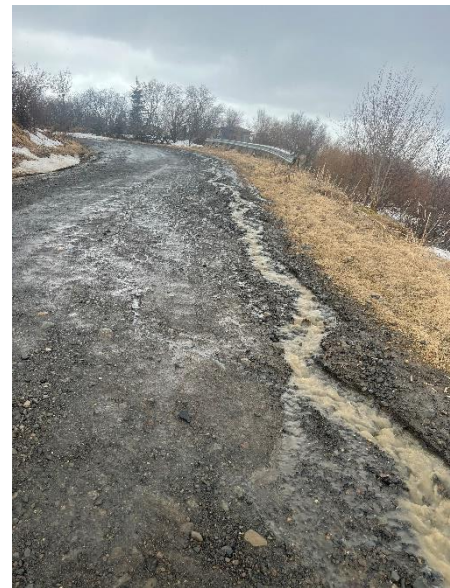
7 Road wash occurring at bottom of hill
