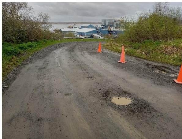
Soft spot with different view
