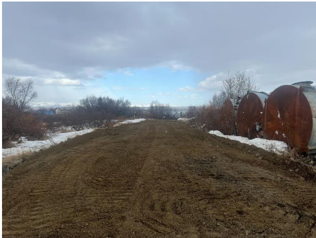
10 Eliminate berm add fines
