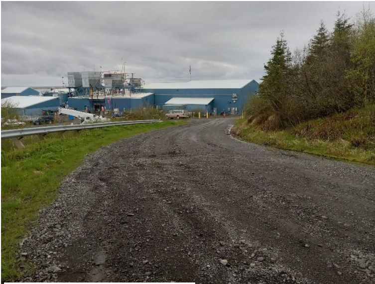
Ditching that needs improvement
