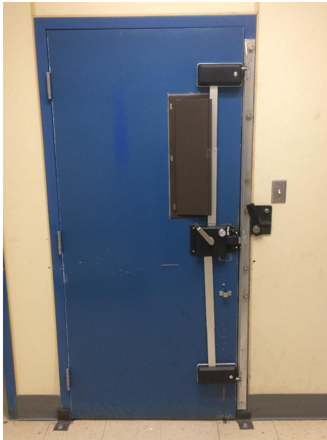
Cell 5 door with new robust security locking system.
