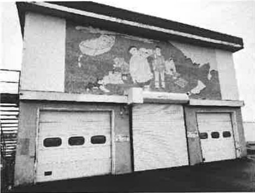
Figure 1: Downtown Fire Station, apparatus doors
