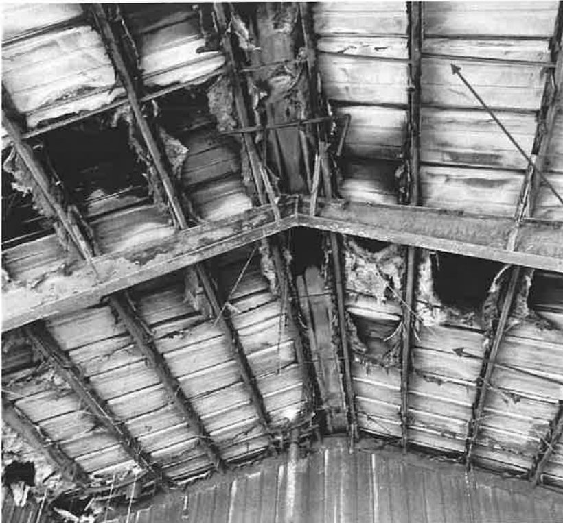
Figure 3: Roof purlins. Bracing indicated
