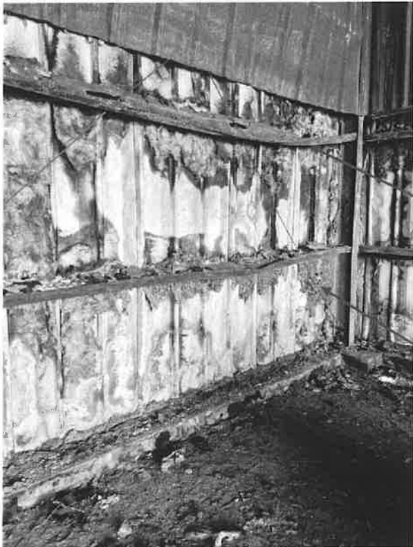
Figure 2: Incinerator building, damaged Z-girts
