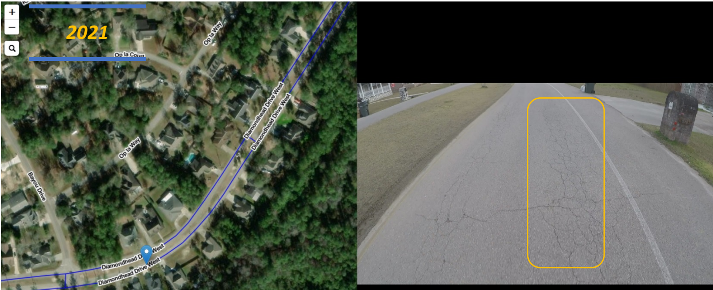
There is significant mass cracking and fatigue cracking along the area between Bayou Drive and 85553 DH Drive West. However, these issues were present in 2019 as indicated in the rectangular areas.
