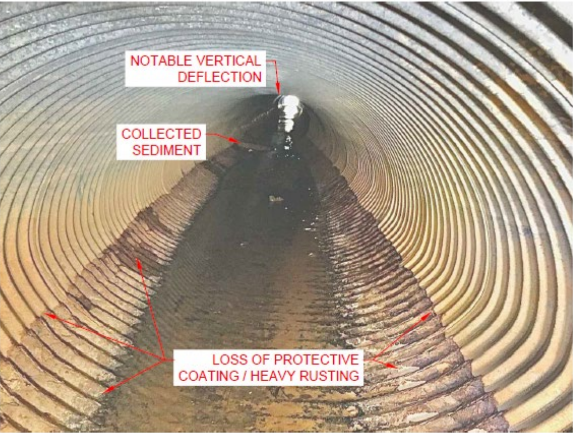
LOOKING UPSTREAM ON UPSTREAM CULVERT
