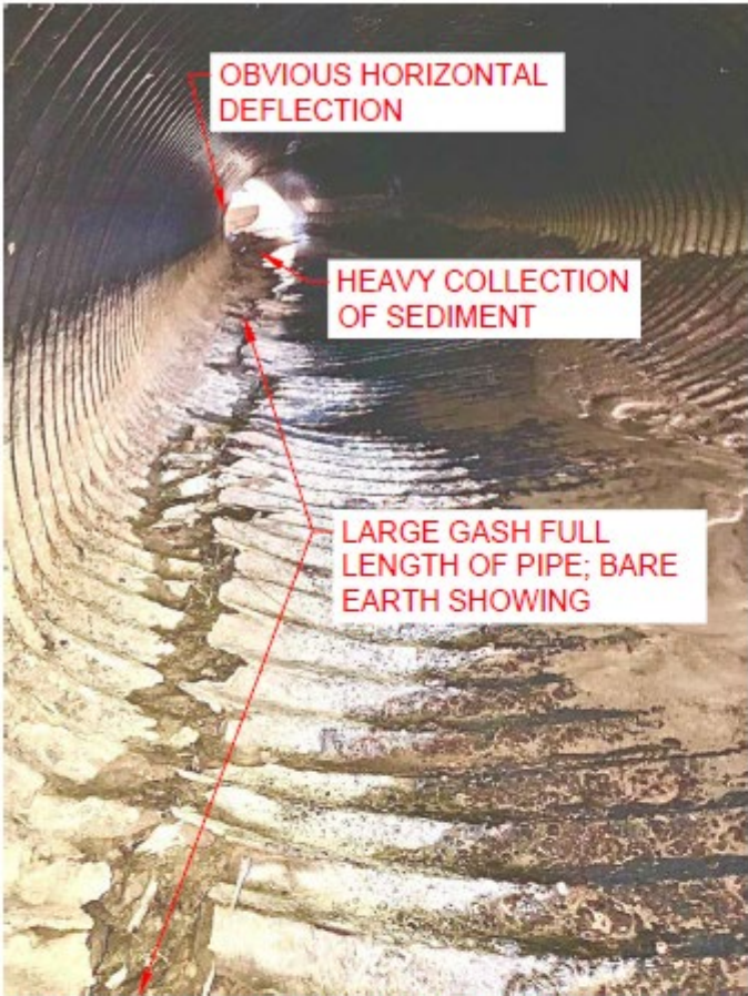
LOOKING UPSTREAM ON DOWNSTREAM CULVERT
