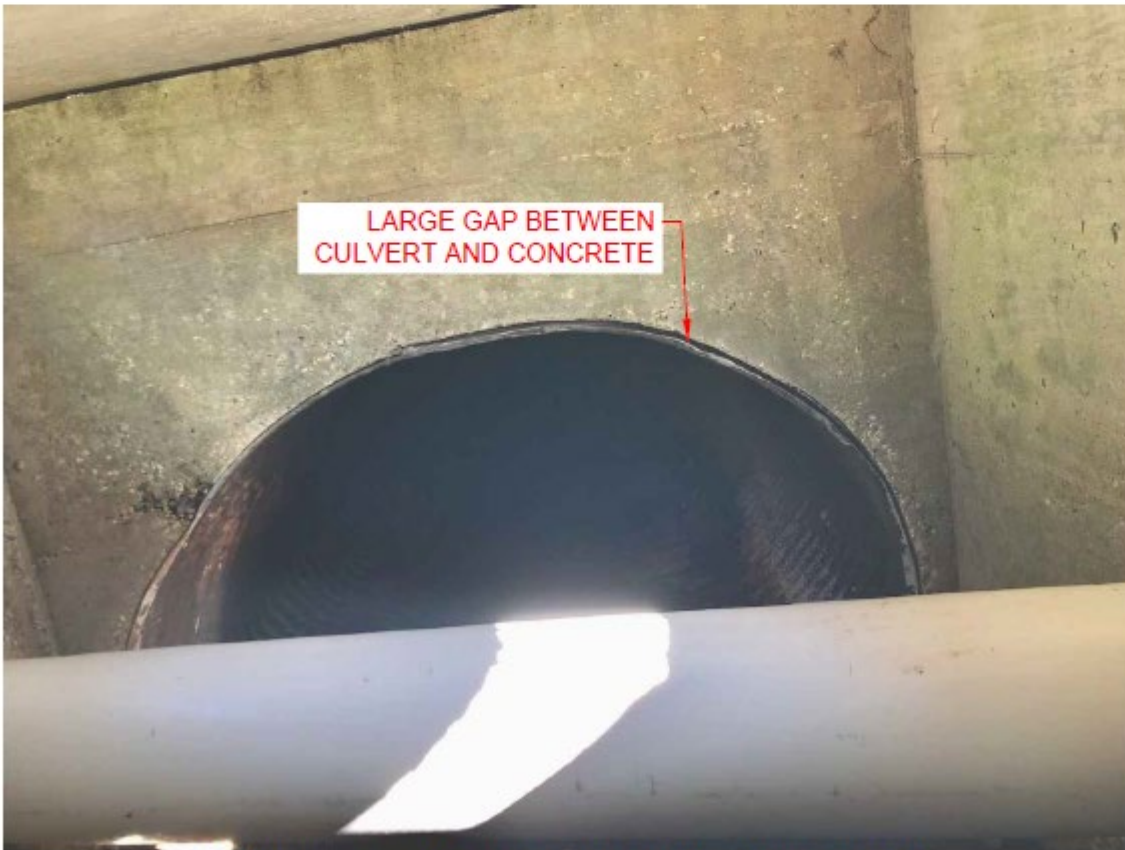
INTERIOR OF JUNCTION KING DOWNSTREAM
