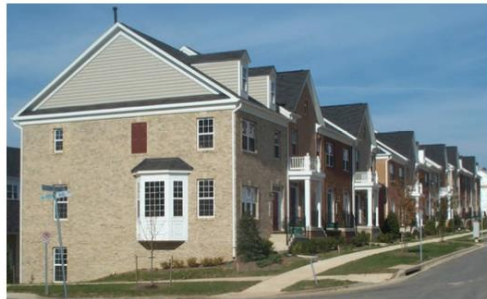
Figure 2.1 Townhouses Townhouses are single family units arranged horizontally in a linear pattern. While the units are attached, each individual unit maintains a private entrance on the exposed front and rear wall of the structure.
