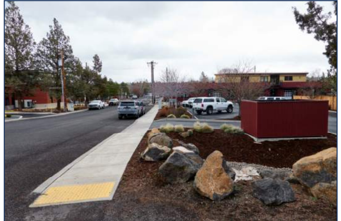
Looking at east sidewalks on 4th Street east of the downtown core.
