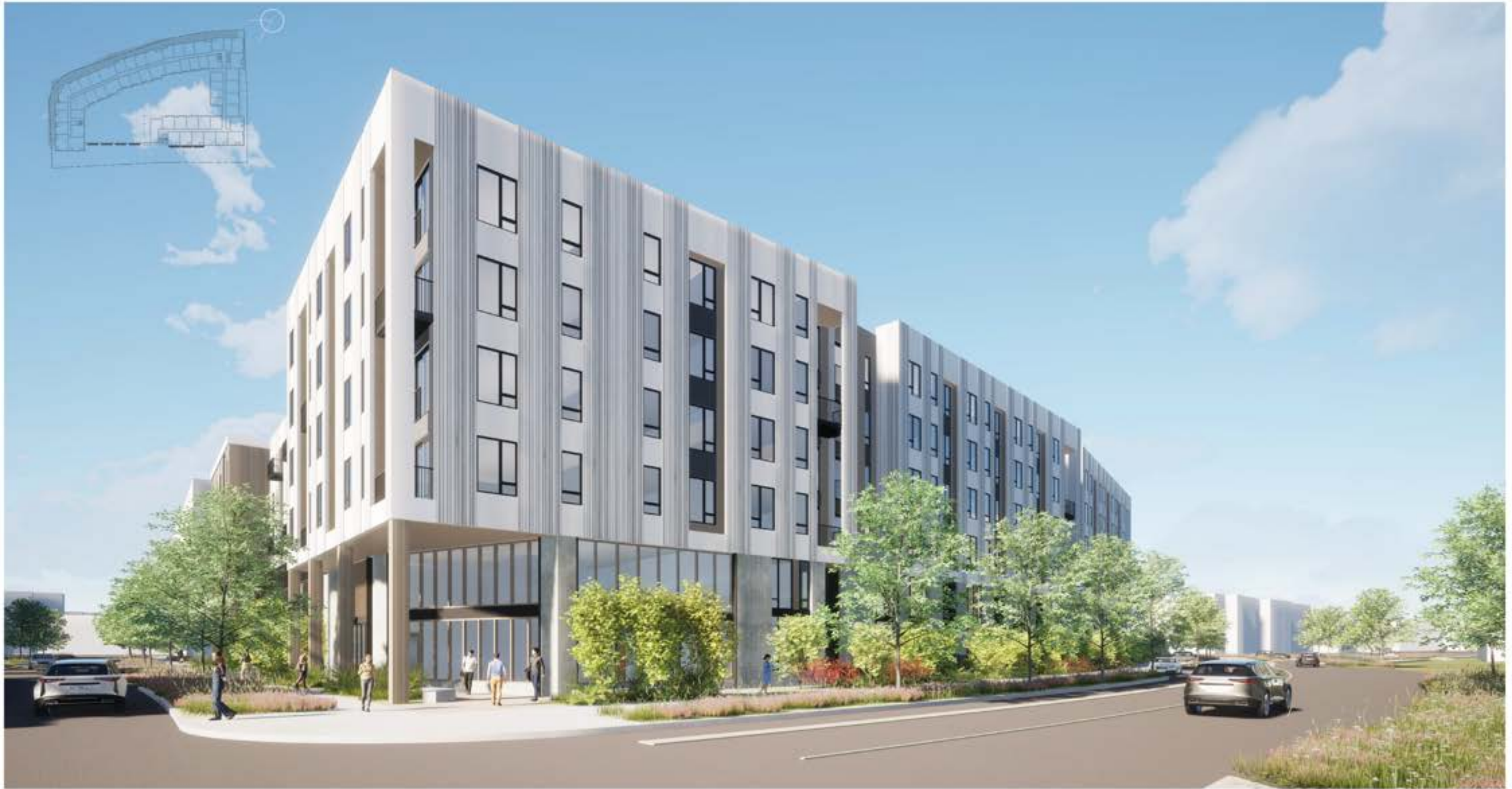
View Looking Southwest Towards Main Residential Lobby Entrance
