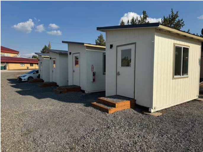
Units at Community Presbyterian Church are 4 of 26 placed between Redmond & Bend
