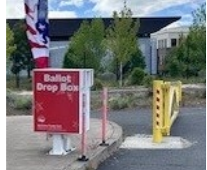
Figure VII: Photos of drop boxes with openings above 48" and gaps wider than ½"
