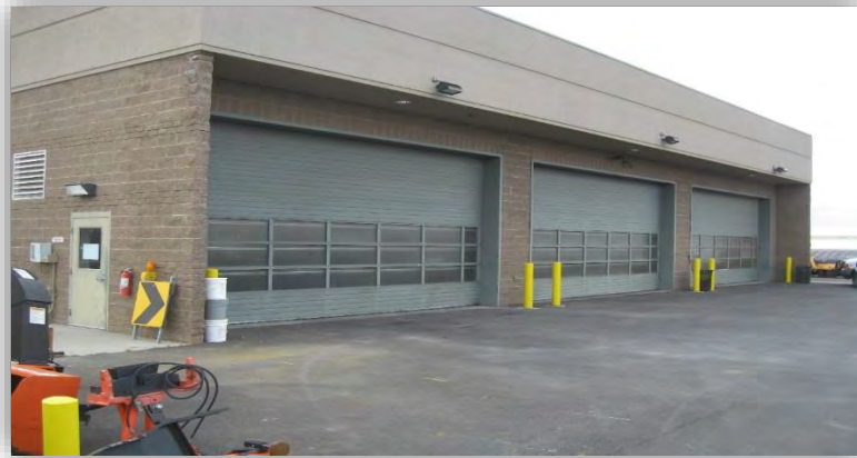
Figure 1-7. SRE and Maintenance Support Facility
