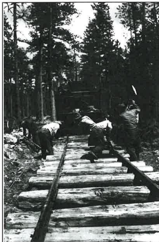
Figure 2 US forest service photo of crews laying track south of Bend.
