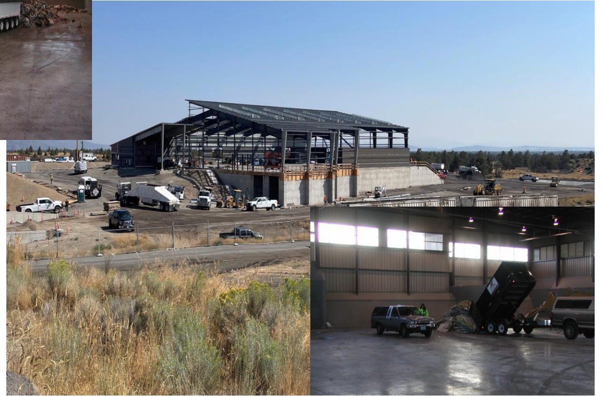
Negus Transfer Station Improvements
