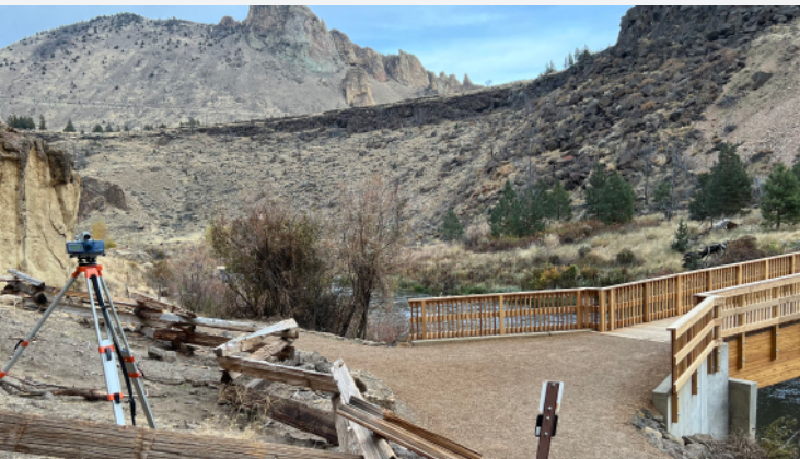
Smith Rock State Park Pedestrian Bridge
