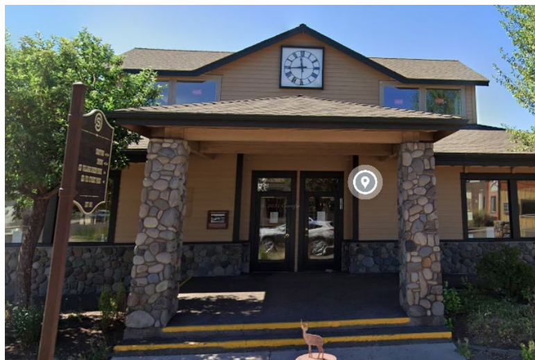
Figure 9: Stone columns and wainscotting used on the covered walkway at 161 E Cascade Avenue.
