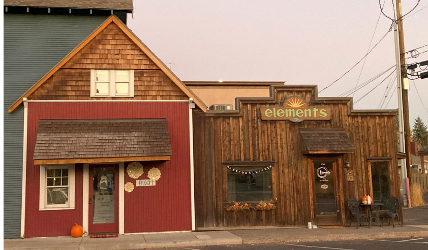
Figure 2: Example of wood shingles used at 130 S Elm Street. These building facades are incorporated into the southside of the “Palace Hotel” building located at 101 E Cascade Avenue originally built in 1915, which is listed on the local historic register.
