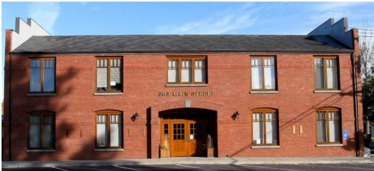
3. Brick Masonry siding used on the 301 E Main Avenue building.
