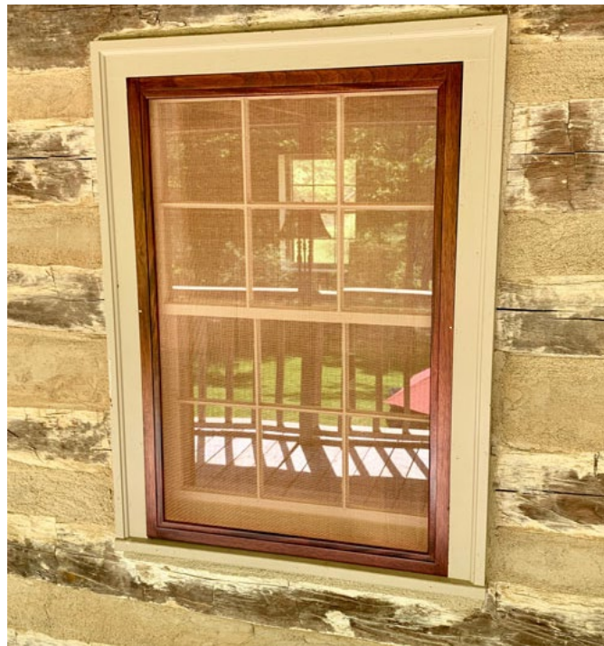
Figure 10: Example of a window screen placed over an old window or historic “glazing”.
