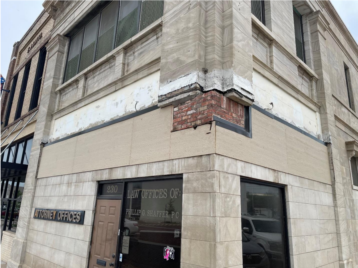
Photo 1, temporary sealing of the removal areas.
