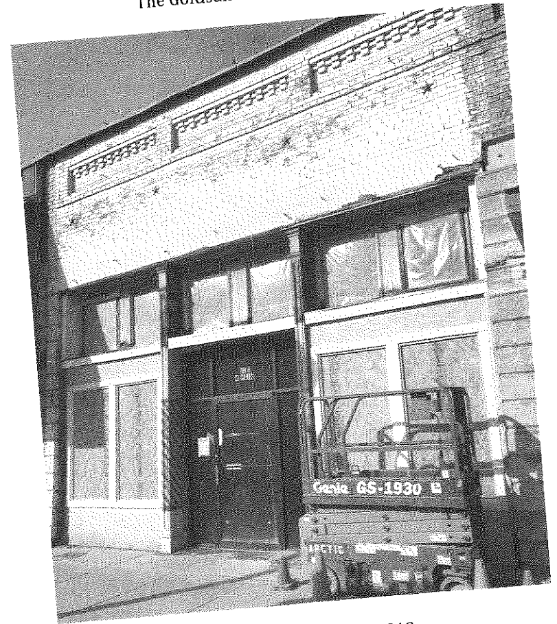
The Goldsall Building, 2019
