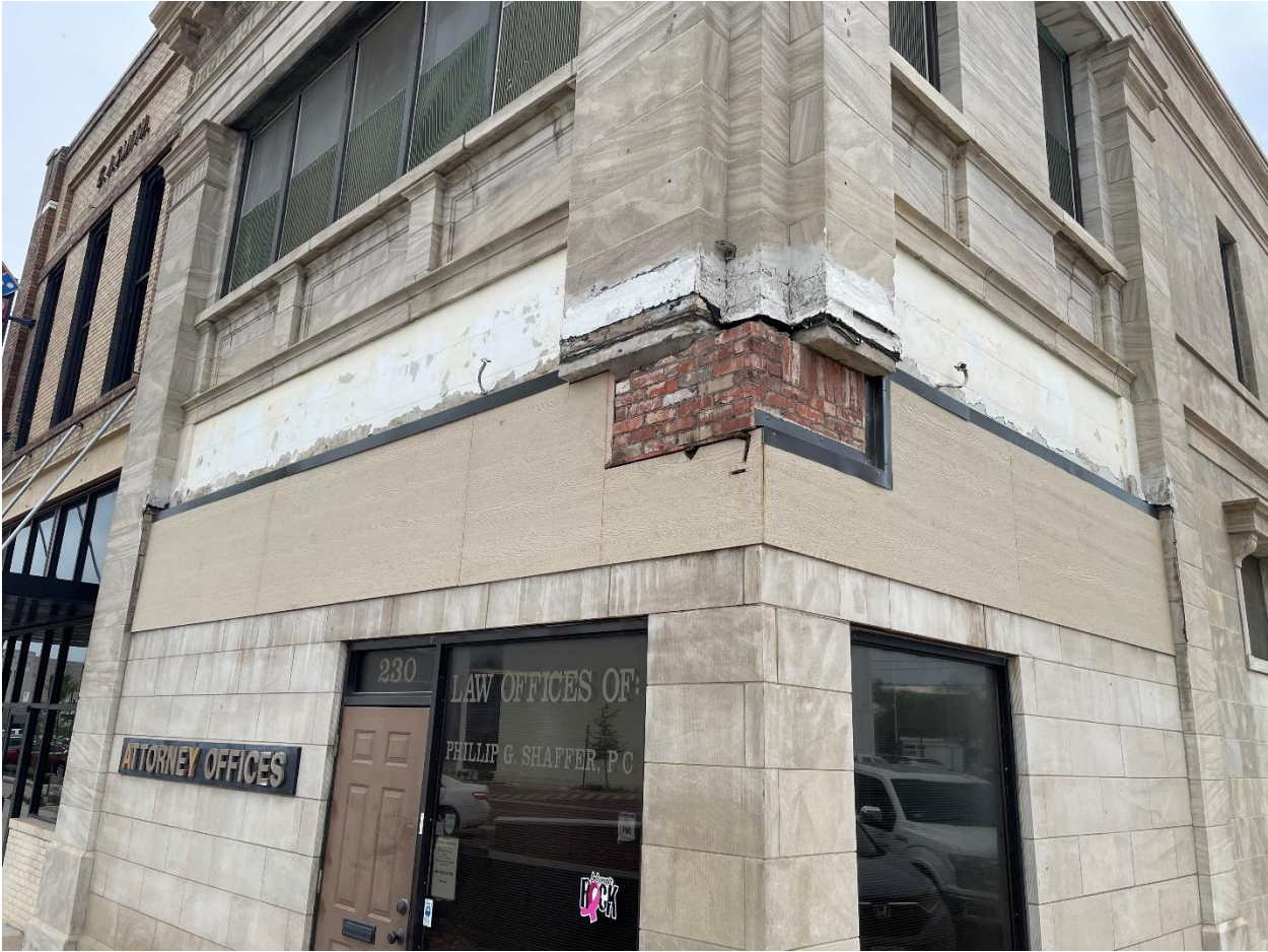
Photo 1, temporary sealing of the removal areas.
