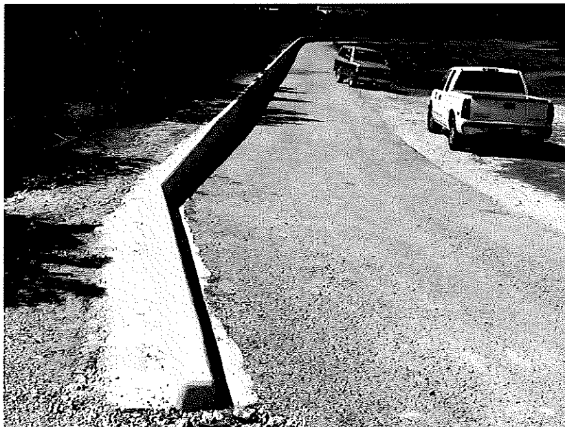
Figure-2: Parapet wall constructed for central Texas dam.
