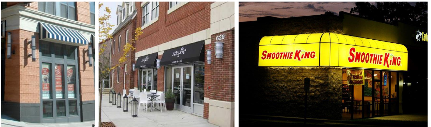
Left: awning installed too high; Center: Awning not deep enough; Right: Backlit awnings are not allowed
