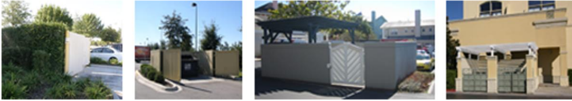
Figure 5 - 76: Screening of Trash Containers
