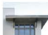
Cantilevered roof planes
