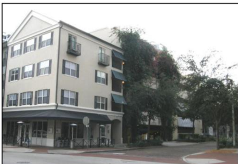
Parking structure behind liner building
