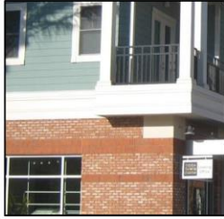
Brick and siding
