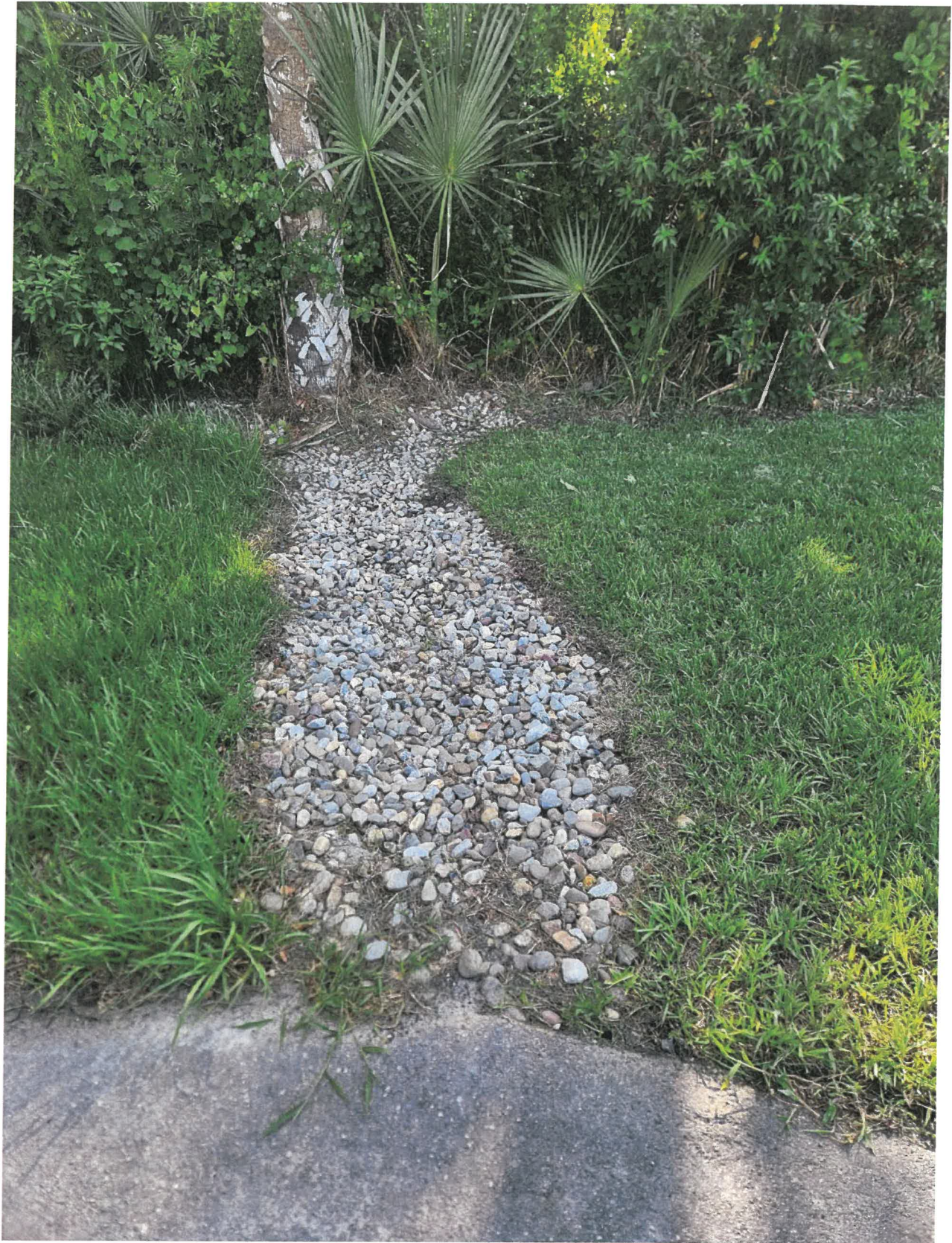
Gravel installed seemingly to minimize wash out and direct water to wet lands.
