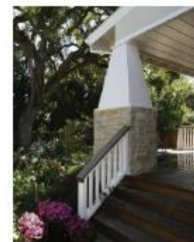
Stairs lead to porch
