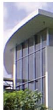
Large glass openings
