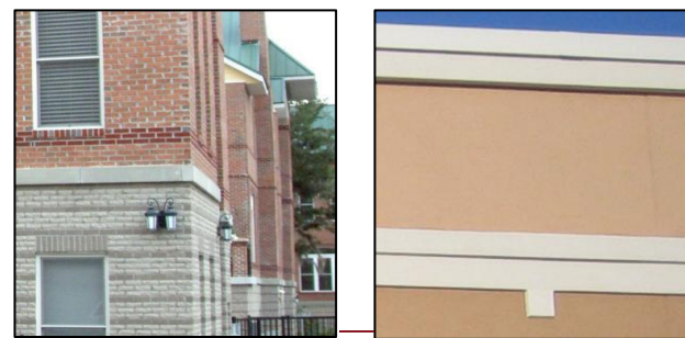
Stone and textured stucco Brick and siding Various bricks Textured stucco with E.I.F.S.
