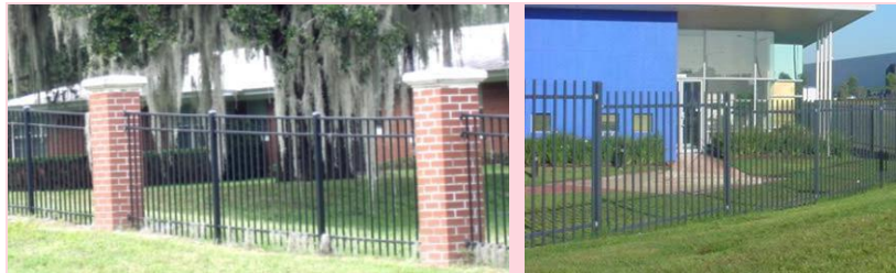
Metal picket fencing alongside/rear yards
