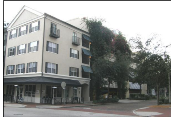
Parking structure behind liner building
