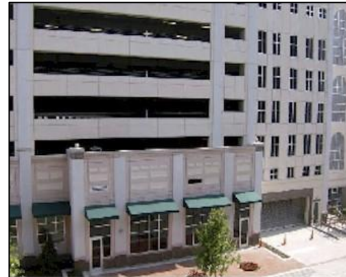
Liner building incorporated into parking structure
