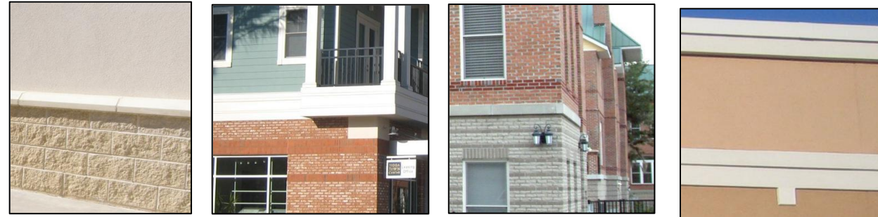
Stone and textured stucco Brick and siding Various bricks Textured stucco with E.I.F.S.
