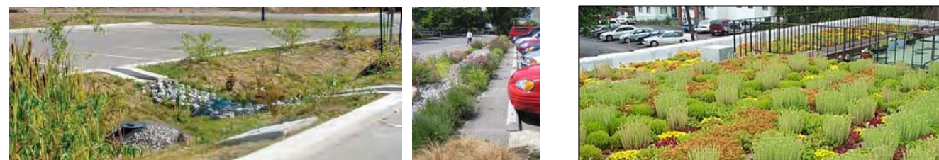
Figure 14: Green Infrastructure [CS3]
