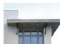
Cantilevered roof planes
