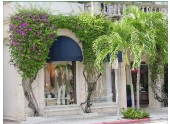
Figure 5 -45: Planters Adjacent to Buildings
