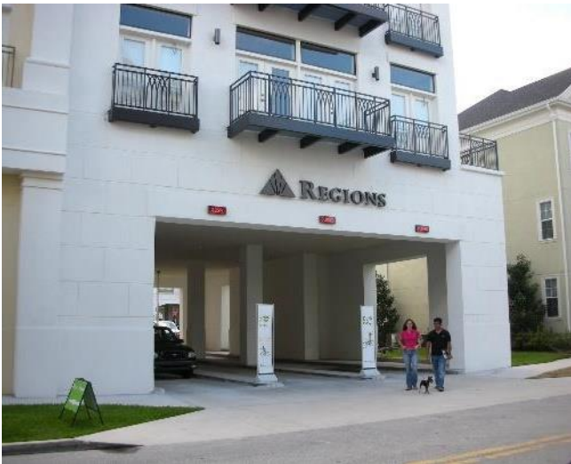
Figure 5 -36: Interior Drive-Through Facilities
