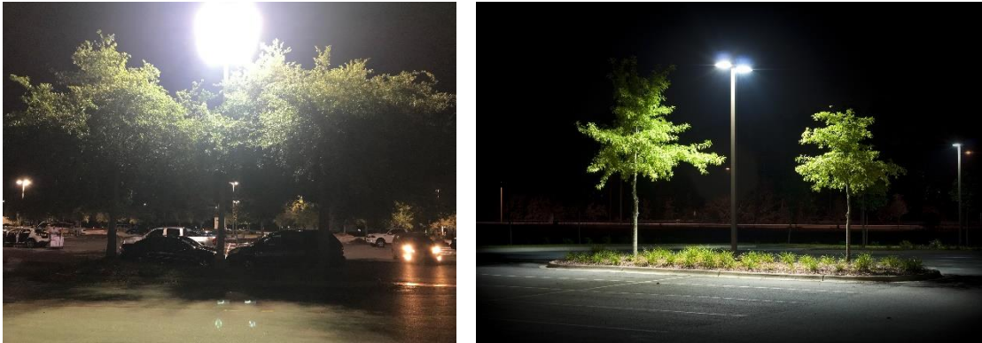
Left: Trees and light fixtures are in conflict; Right: Lights coordinated with trees
