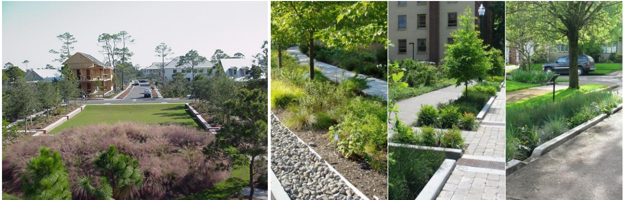
Figure 5 -50. Alternative Stormwater Detention/Retention Facilities
