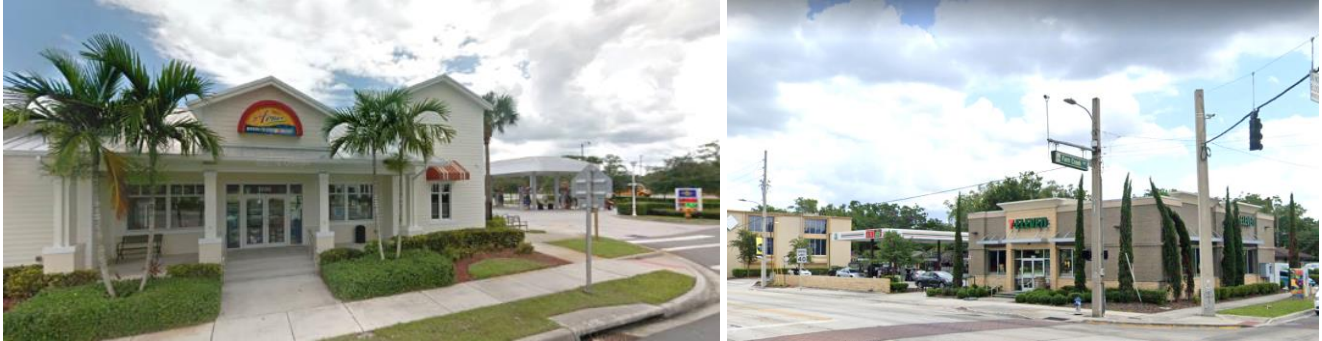
Figure 5 -33: Service Station Examples
