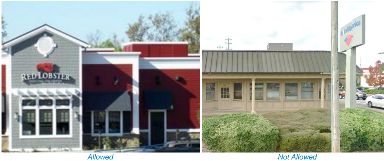
Figure 5 -32: Rooftop Units Screening
