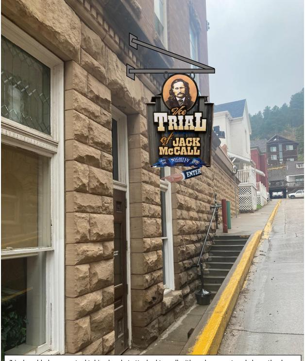
2 inch welded square steel tubing bracket attached to wall with anchors, centered above the door.
