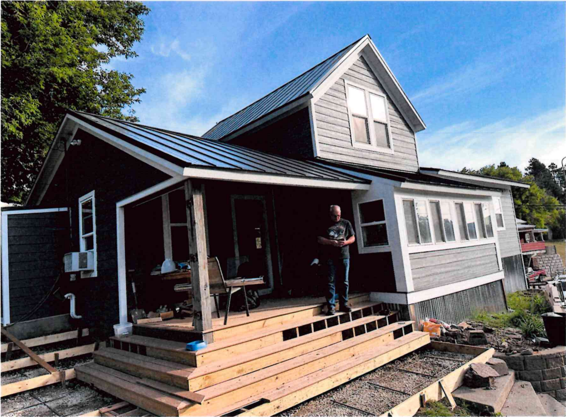
EXAMPLE - HOUSE JUST COMPLETED IN LEAD
