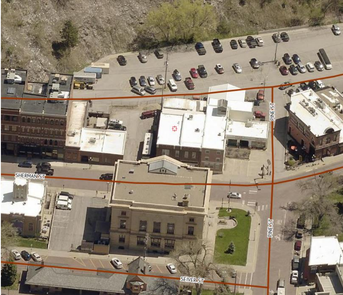
Aerial photo of 65 Sherman Street, Deadwood, SD 57732.
