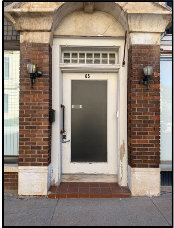
65 SHERMAN EXISTING FRONT DOOR
