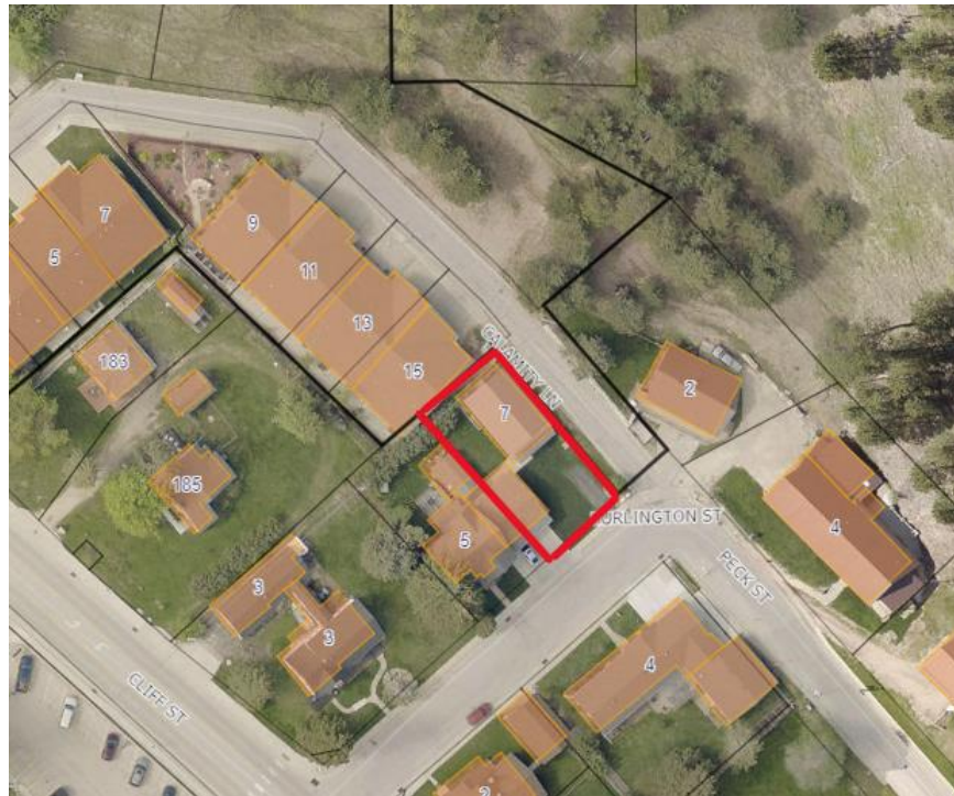
Aerial photo of 7 Burlington Street
