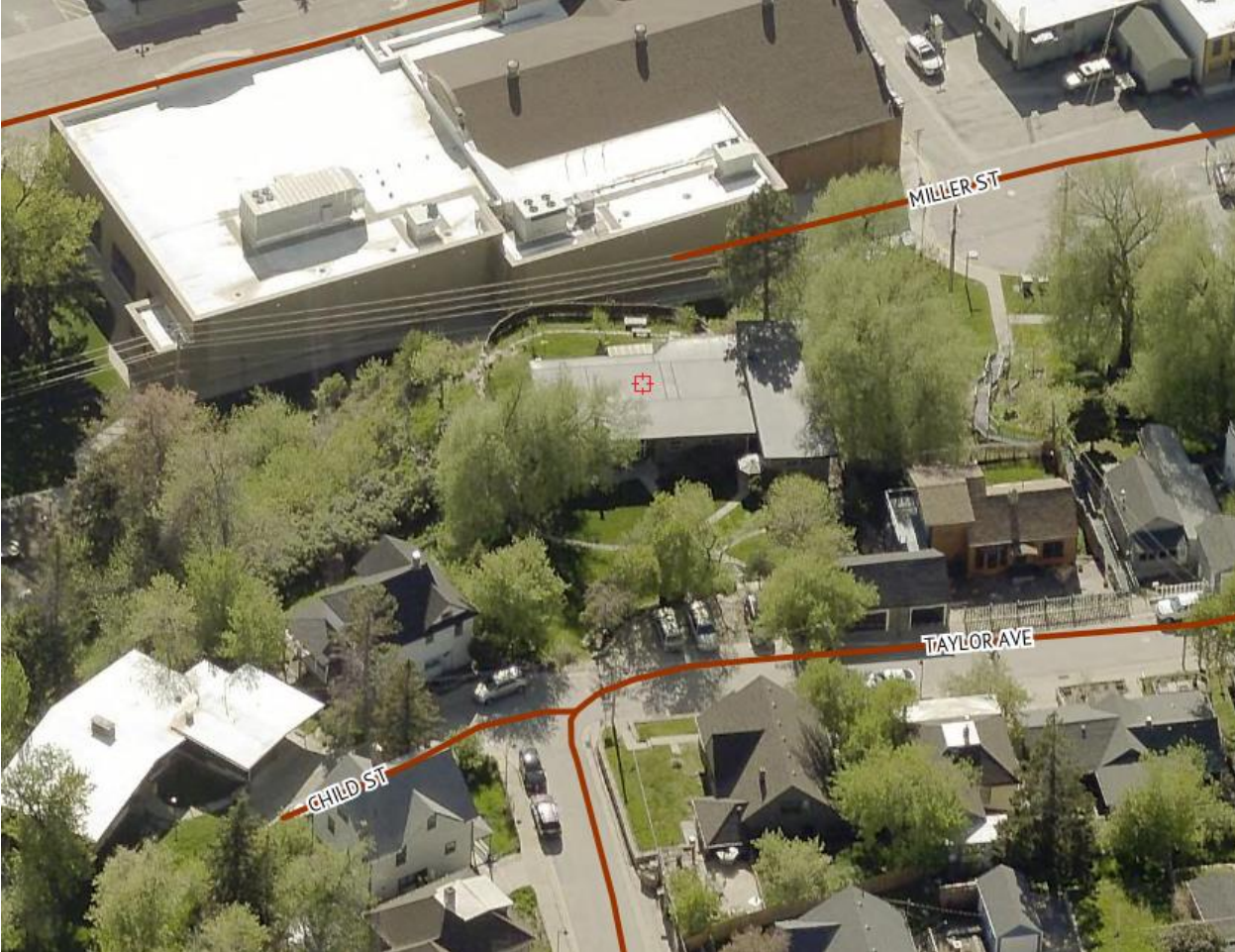
Aerial photo of 56 Taylor Avenue, Deadwood, SD 57732.
