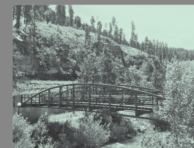
Bridge Over Whitewood Creek
